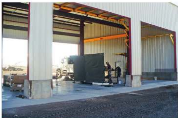
A new shop allows mechanics to stay out of the hot Arizona sun while performing maintenance and repair on equipment, which is important since the Queen Creek operation handles the maintenance for all of its operations.
